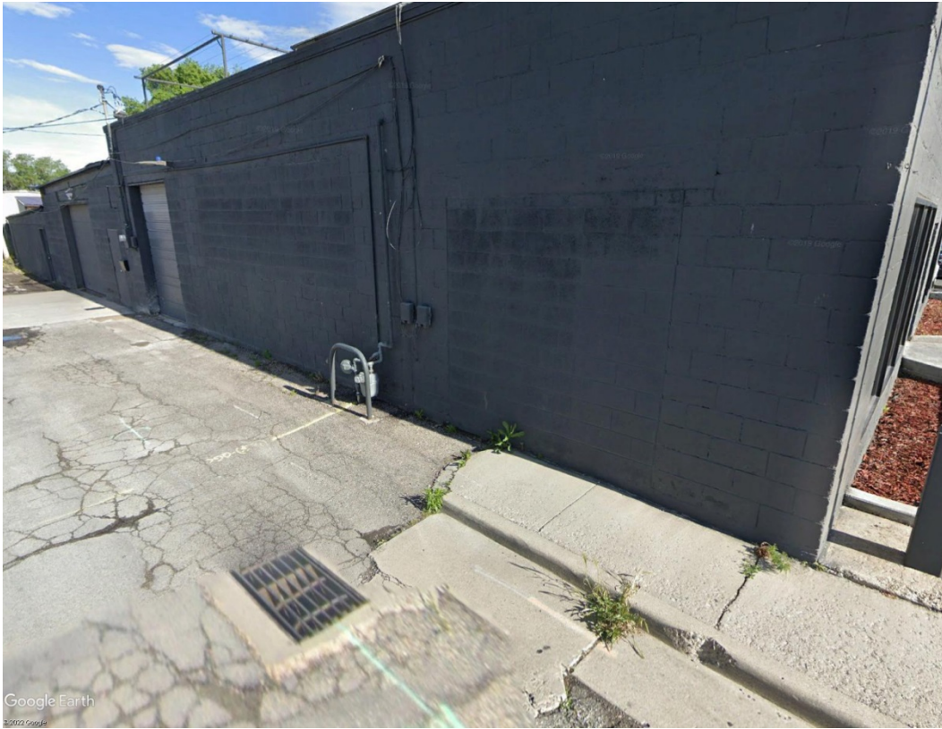
Rev Motoring Already built to sidewalk on Andrews Street
