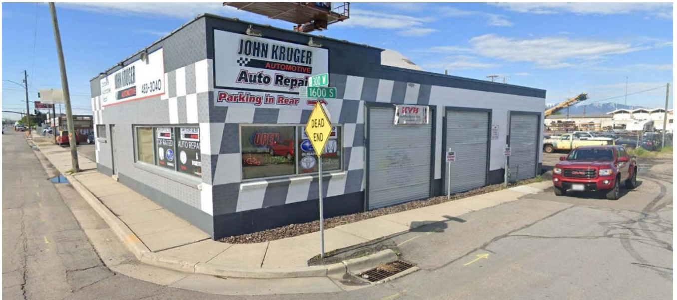
John Kruger Auto Repair located at 1604 S 300 W built up to the sidewalk
