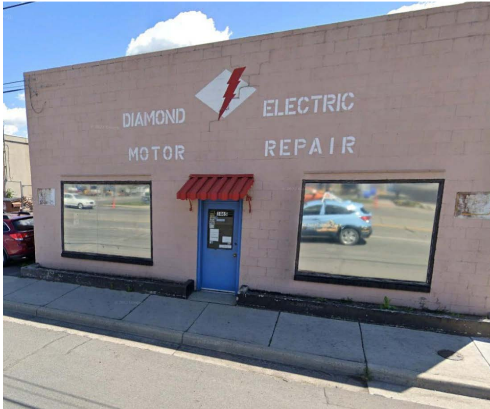
Diamond Electric located at 1465 S 300 W built up to the sidewalk
